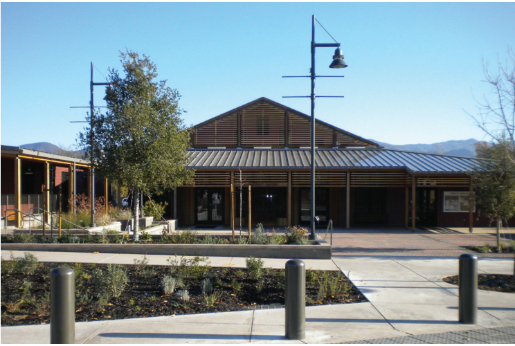
PROJECT: Yountville Community Center - Yountville, CA ARCH: Siegel & Strain LT DES: Alice Prussin Lighting Design SPEC Nos: 3D-2352 Pendant; 1D-2352 Ceiling (2009)
